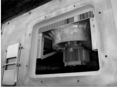
b) Loosen 4 pcs bolts (M8) from fan blade fixing metal.
