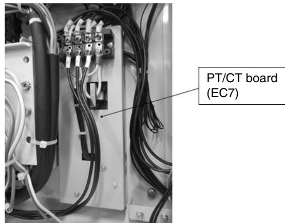
This printed circuit board has the two functions as a measuring instrument and protective device and provide as an interface between the main circuit (high voltage) and controller.
